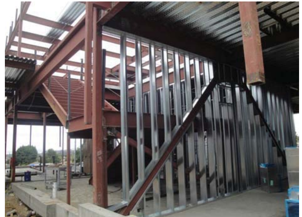
Building C - metal stairs and metal framing
