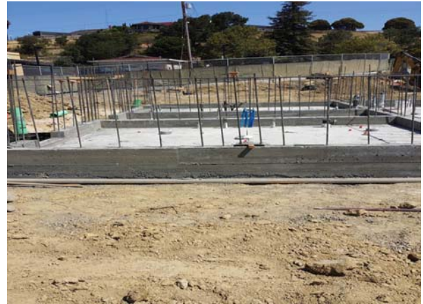
Soccer Field - Concrete Slab & Curb @ Restroom Building
