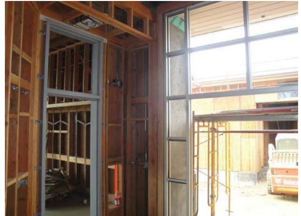
Building A - Door and storefront framing
