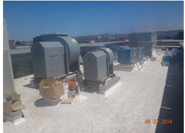
Building A - Mechanical units and ductwork at roof area
