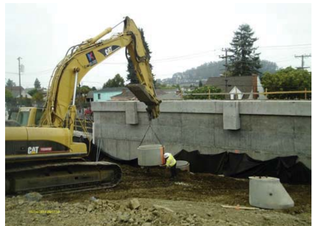
Central portion of Ashbury Retaining Wall manhole
