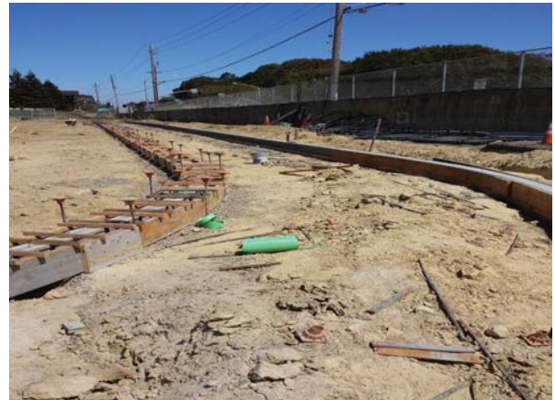
Soccer Field - Perimeter trench drain and curb @ track
