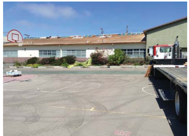
Building A - Installing Waterproof Membrane
