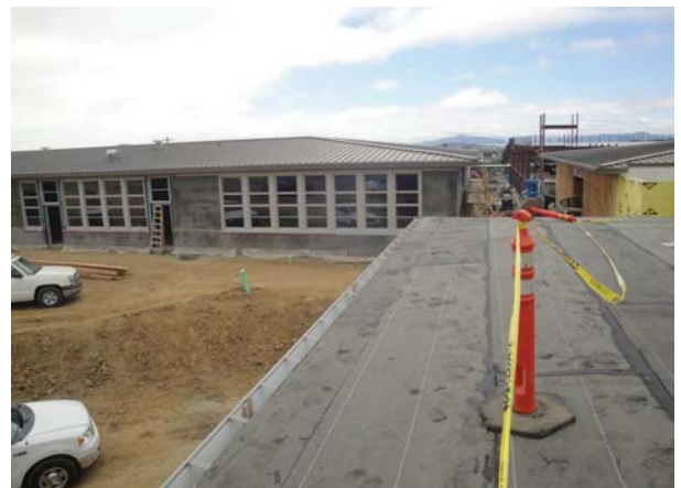
Building A - Windows and Building D- roof installation
