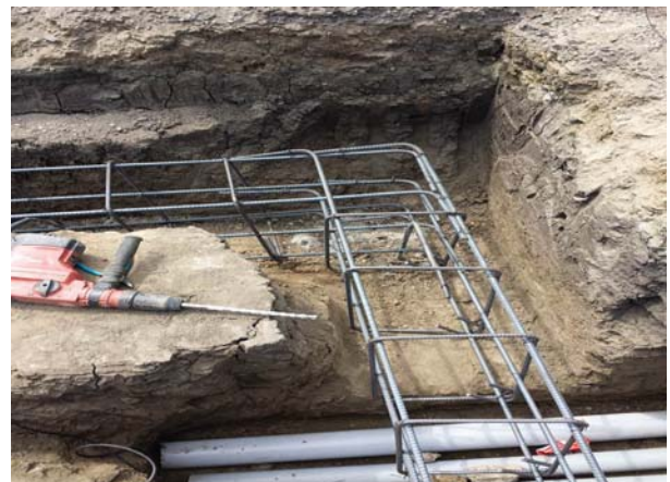
Grade Beam Rebar installation & Under Ground Electrical
