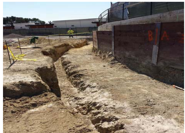
Soccer Field -Retaining Wall Footing Excavation
