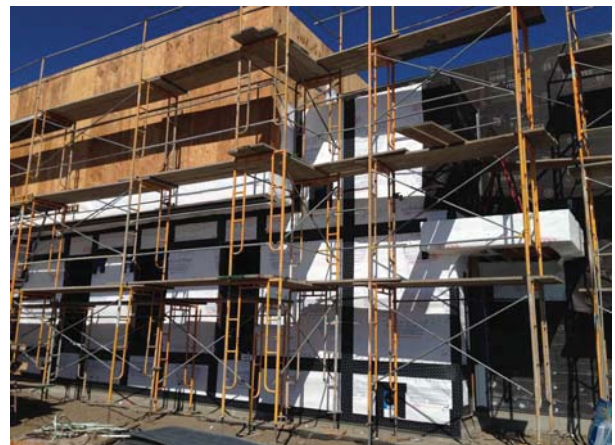
Building M Scaffolding Erection (Plaster)
