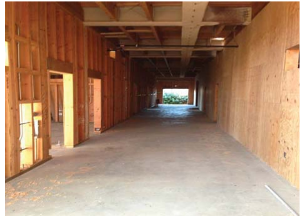
Building C Corridor (Interior Ply Framing)
