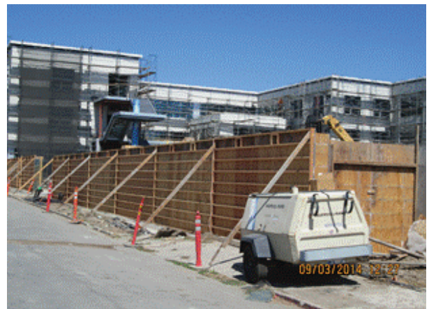
Site: Wall formwork at west side.
