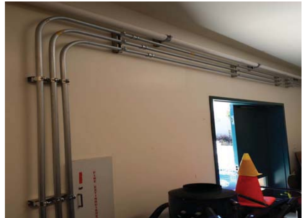
Interior Electrical Conduit Installation in Mechanical Room
