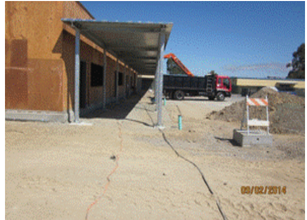
Structural steel, metal decking & covered walk way
