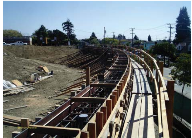
Ashbury retaining formwork for concrete pour
