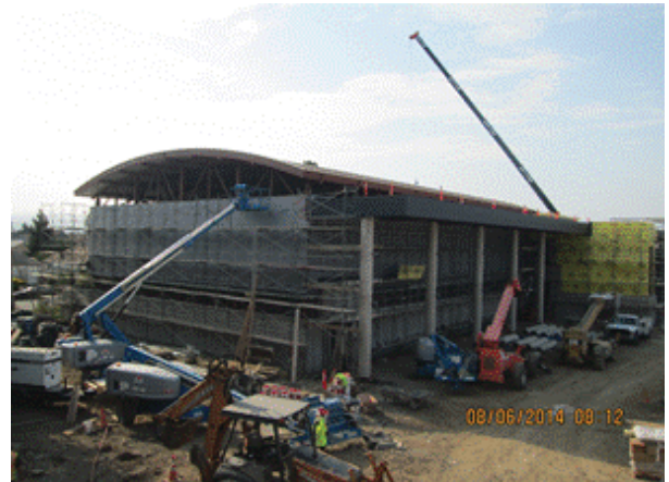
Building B - Gym: Crane setting HVAC units on roof.
