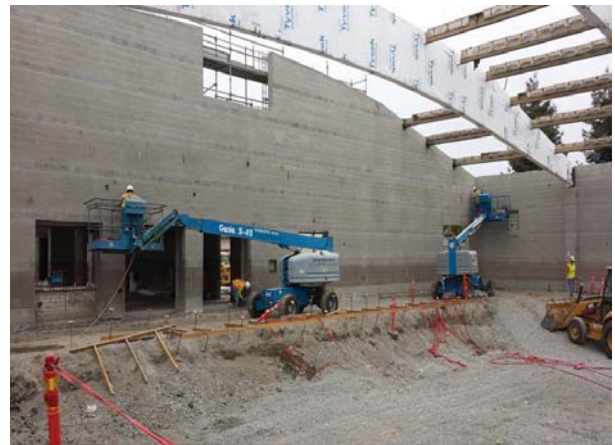
CMU Surface grindings
