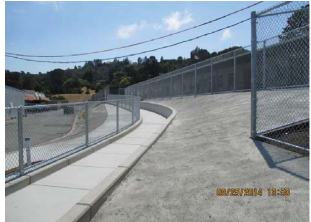
New Walkway Ramp
