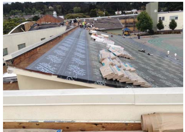
Building A-1 South Roof - Installing Waterproof Membrane
