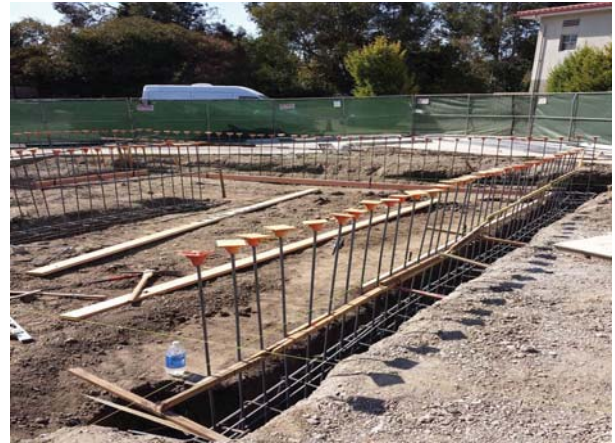
CMU Rebar Installation
