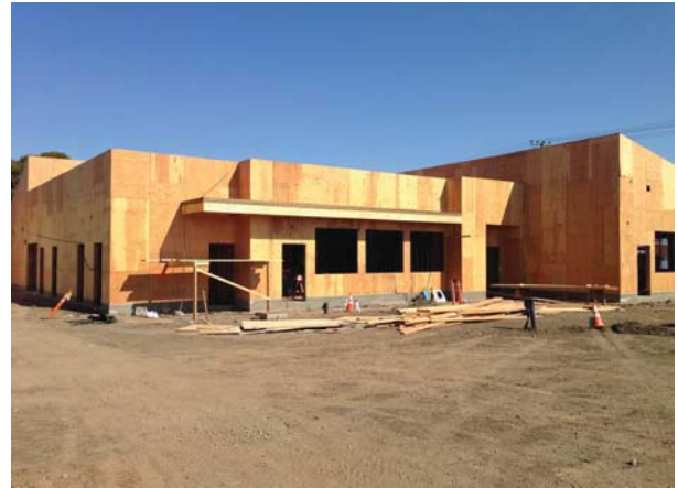
Building K Exterior Framing
