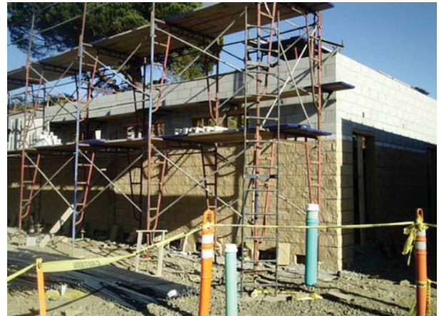
Building D Concrete Masonry Units
